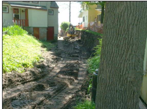
Working between two cottages
